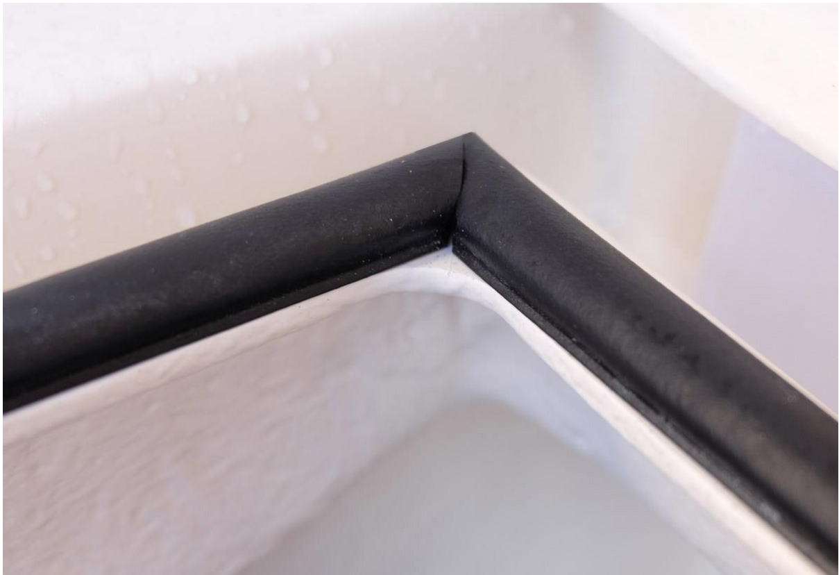
Above: Stop the D-section self-adhesive seal approximately 50mm short of the ends.
